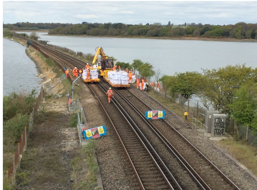
Repairs at Poole Harbour, April 2017
