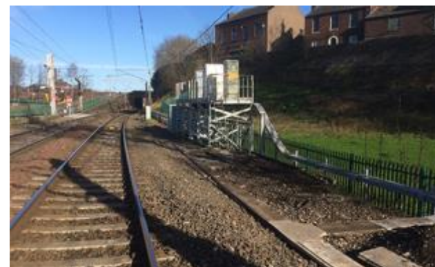
Flood resilience works at Caldew Junction, Carlisle
