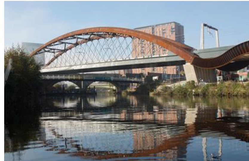
The Ordsall Chord as recently constructed in Manchester
