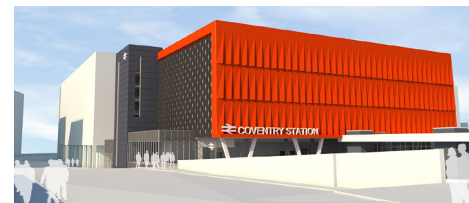
Coventry Station enhancements
