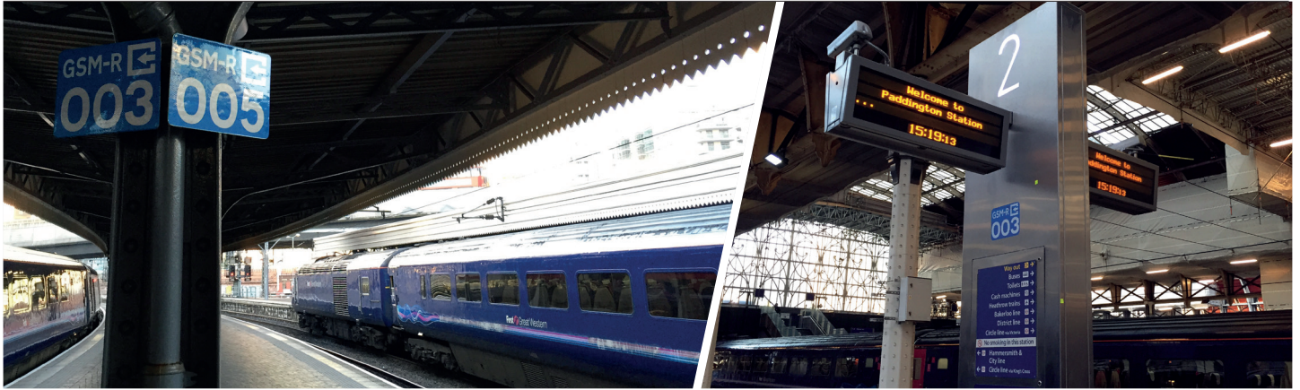
Signs help drivers where signal numbers cannot be seen easily from the train cab
