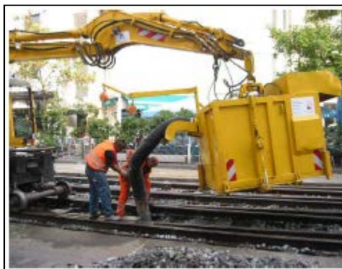
Fig. 9 TubeCube is a road rail vehicle attachment for cleaning ballast
