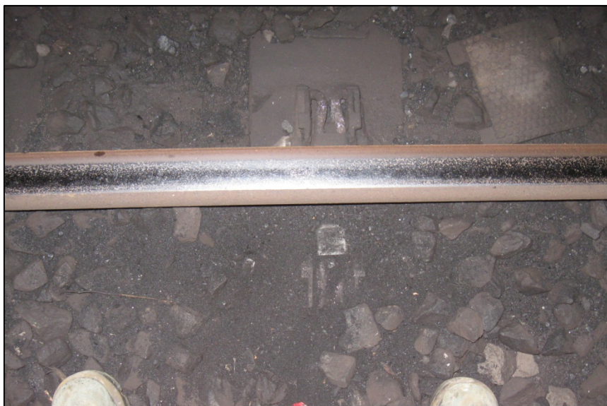
Fig. 6 Plain line in Severn Tunnel
