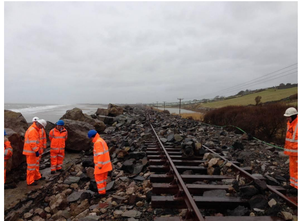
Figure 11 Cambrian Line, Llanaber sea wall, December 2013
