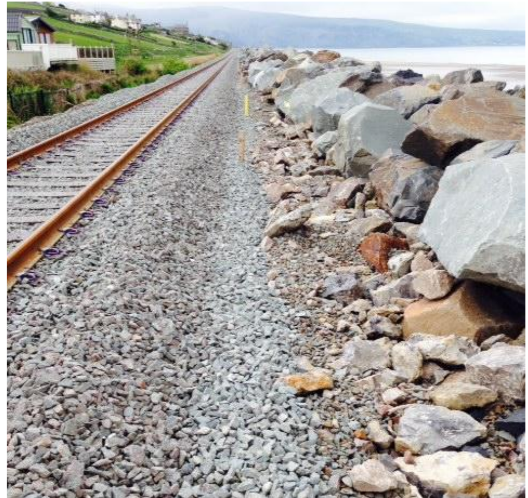
Llanaber following completion of emergency works
