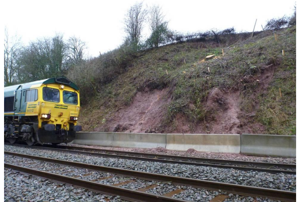
Figure 21 Hereford to Newport Line, Llanvihangel before remediation
