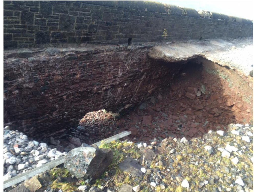
Figure 13 South Wales Main Line, Ferryside St Ishmaels sea wall January 2014
