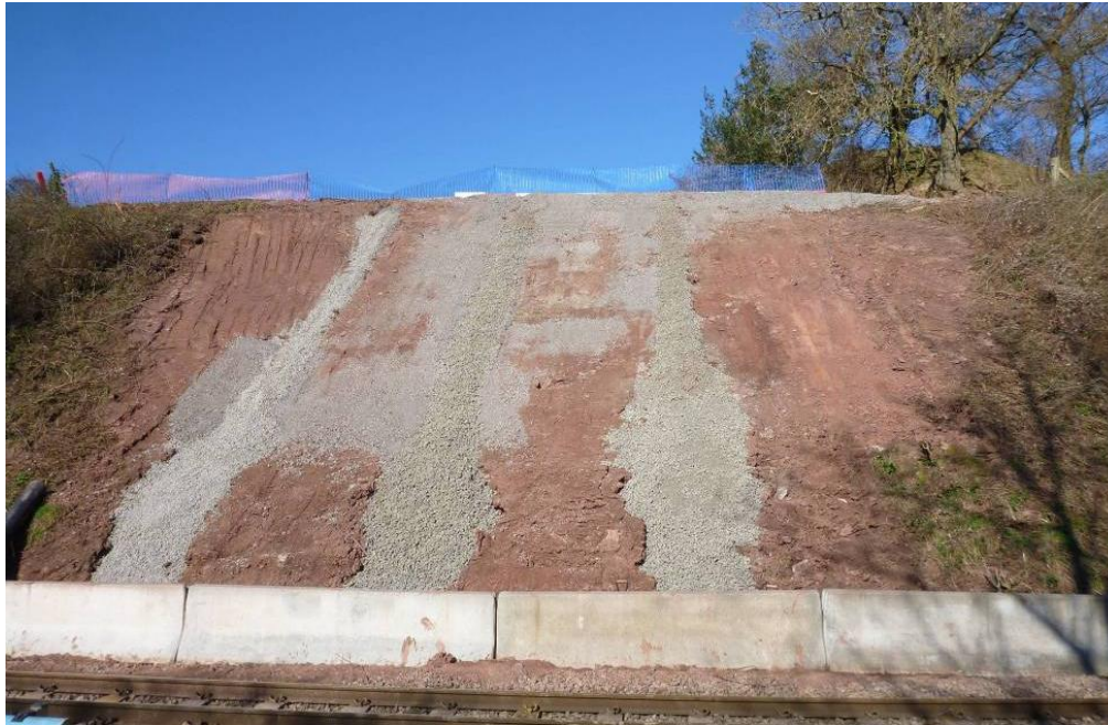
Figure 22 Hereford to Newport Line, Llanvihangel after remediation
