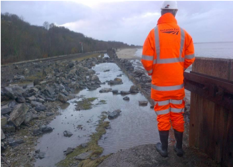
Chester and Holyhead Line, Mostyn sea wall, December 2013
