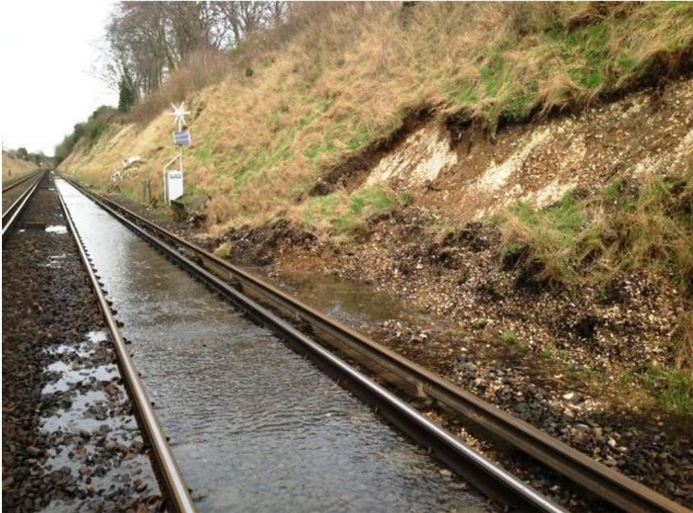
Figure 14 Groundwater flooding at Woodplace, Sussex, in February 2014.
