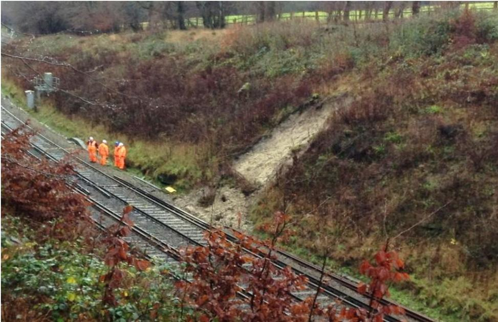
Figure 8 Cutting failure on TTH at Mountfield, Kent, in December led to major slope stabilisation
