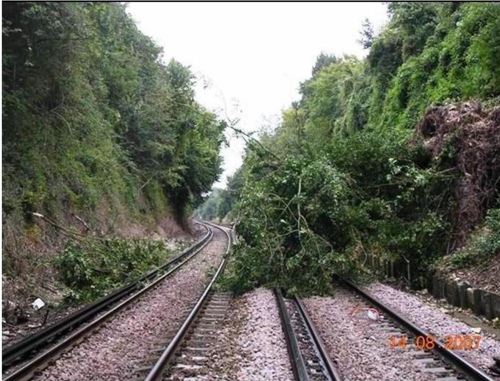
Figure 22 Tree collapsed in the VIR cutting at Sole Street, Kent, in August 2007.
