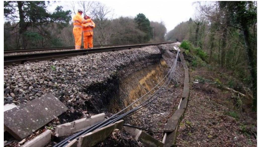
**Figure 24** Embankment failure on BTH at Ockley, Sussex, in December 2014.
