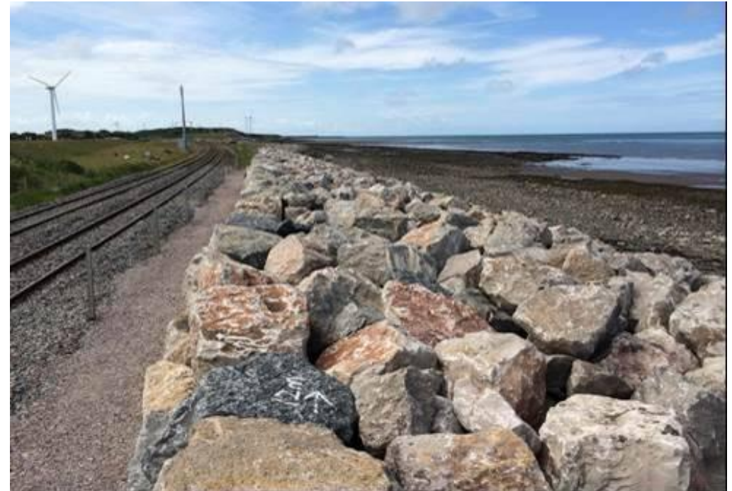
Figure 45 Reinstated sea defence at Siddick sea wall following storm damage in January 2014
