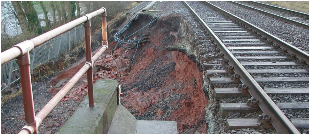
Figure 23 Scour failure on the West Coast Mainline at the River Eden Viaduct
