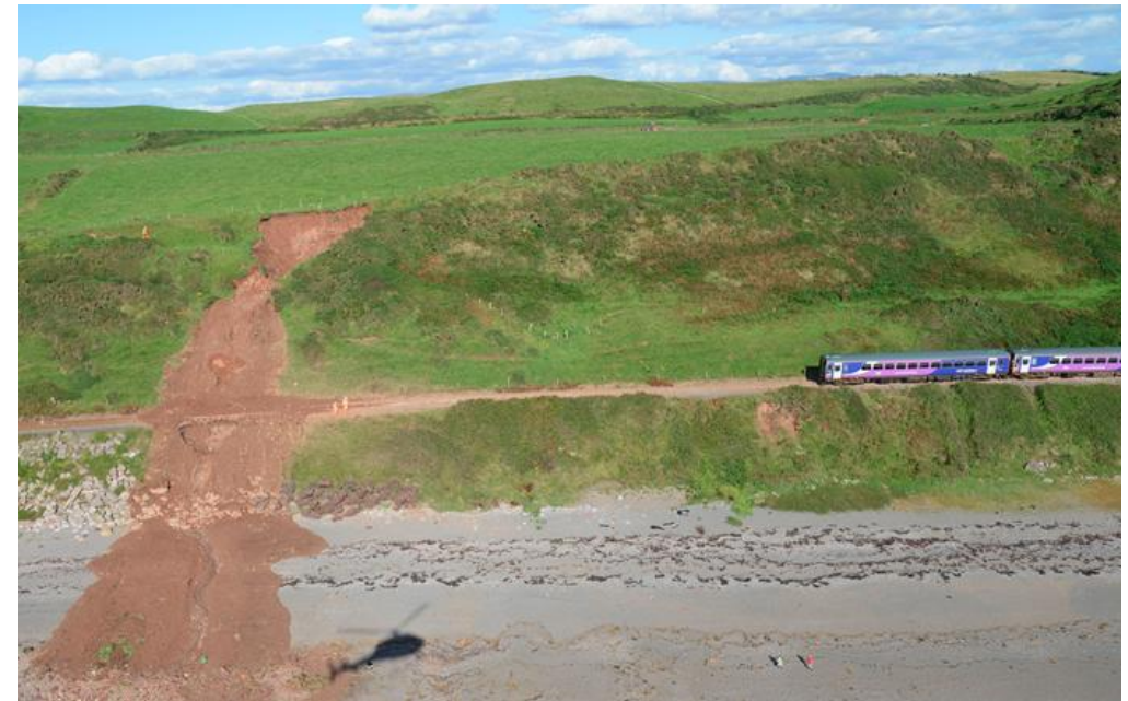
Figure 41 Earthflow failure at St Bees in August 2012
