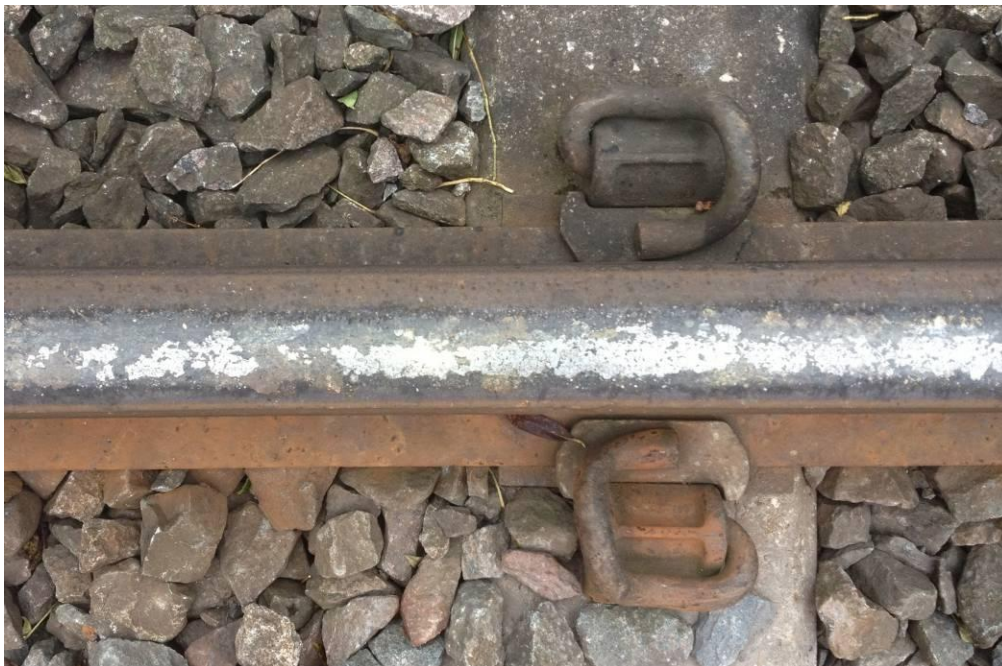
Figure 35 Example of railhead contamination which can cause adhesion issues
