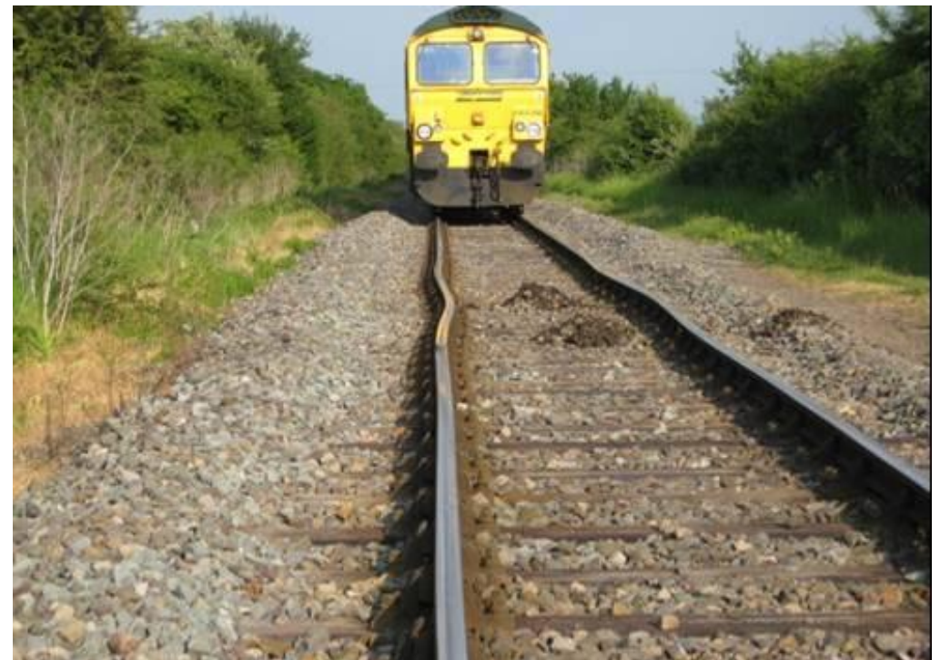
Figure 37 Track buckle at Waddeson near Aylesbury on LNW Route
