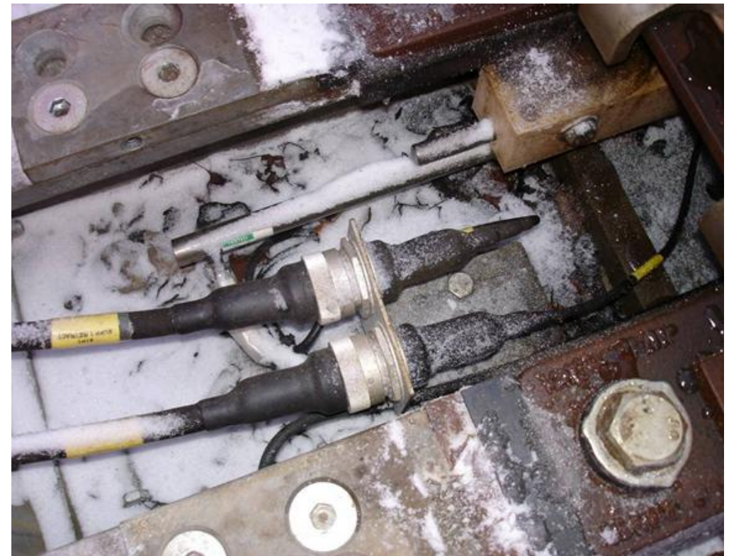
Figure 34 Snow inside point operating equipment
