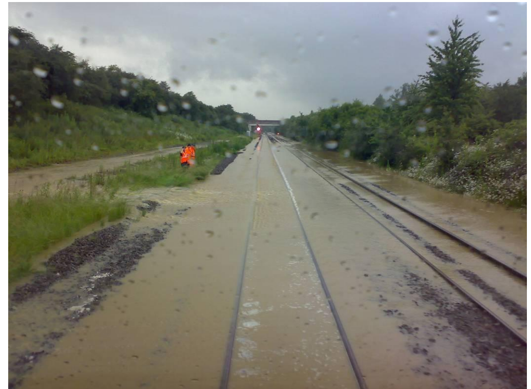
Figure 29 Flooding at Fenny Compton prior to the improvement works carried out in 2013
