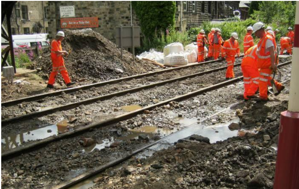
Figure 30 Material deposited on track during flooding at Walsden in July 2013
