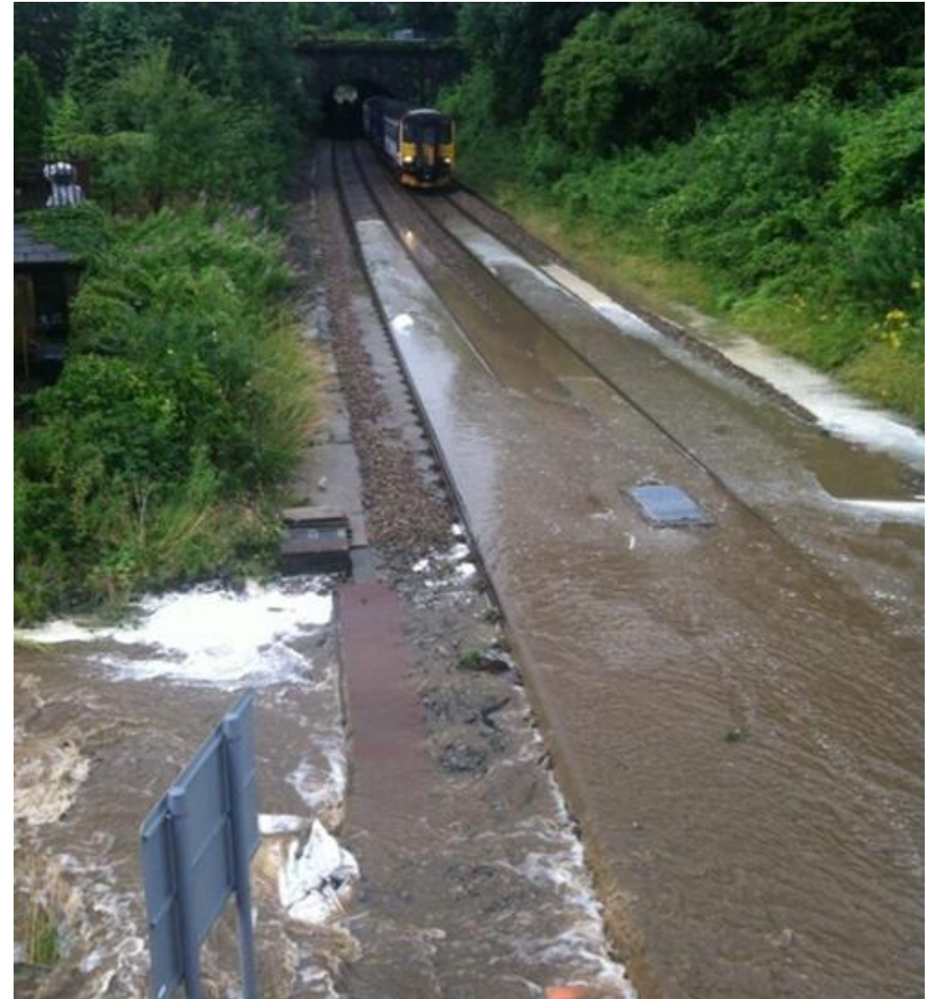
Figure 31 Flooding at Winterbutlee tunnel at Walsden in July 2013 when severe thunderstorms with heavy rainfall caused a third-party upstream culvert burst near Walsden Station resulting in water flowing directly on to the track
