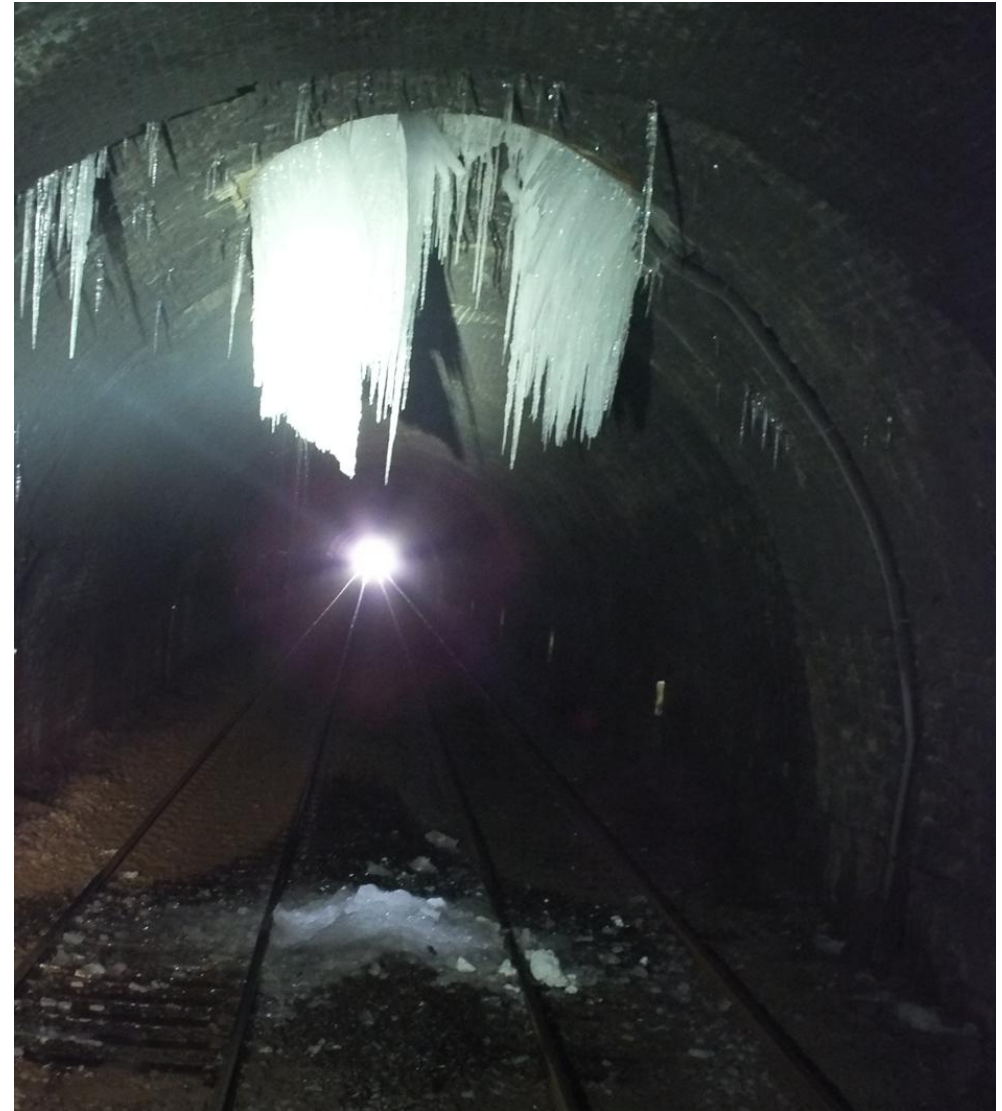
Figure 13 Ice formation emanating from tunnel shaft in Birkett tunnel on Settle to Carlisle railway line
