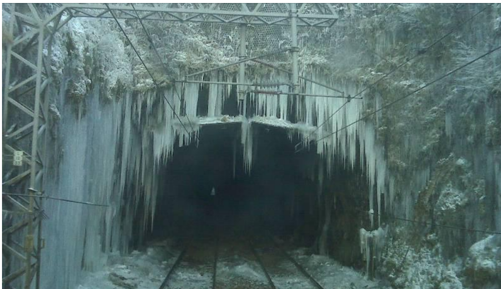
Figure 33 Icicle formation in a tunnel impacting gauge clearance and overhead line equipment
