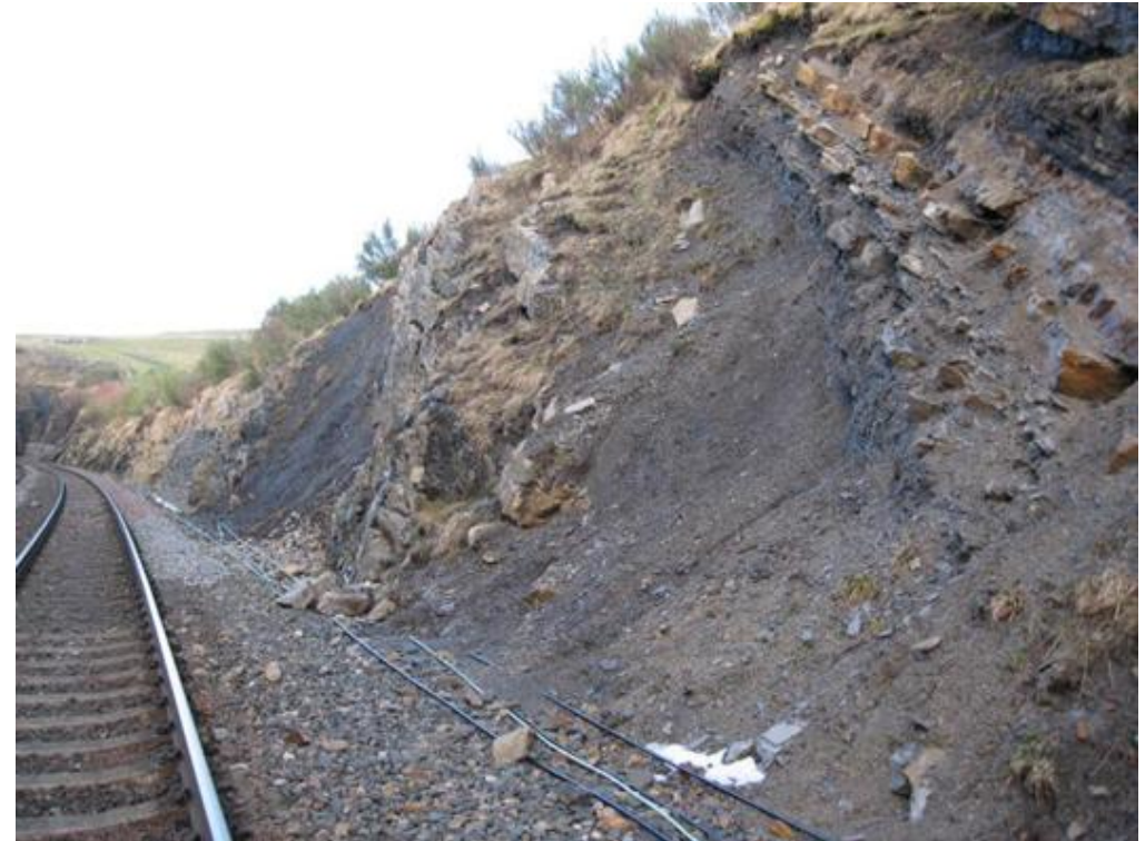
Figure 42 Accelerated weathering of softer rock slopes at Birkett in 2009
