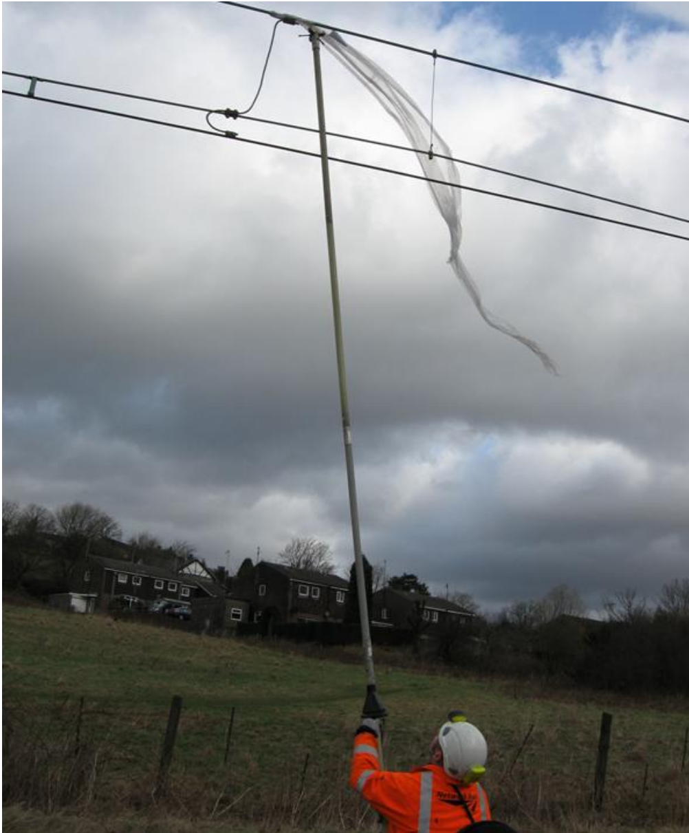
Figure 26 Removal of plastic sheeting from overhead line equipment on LNW Route
