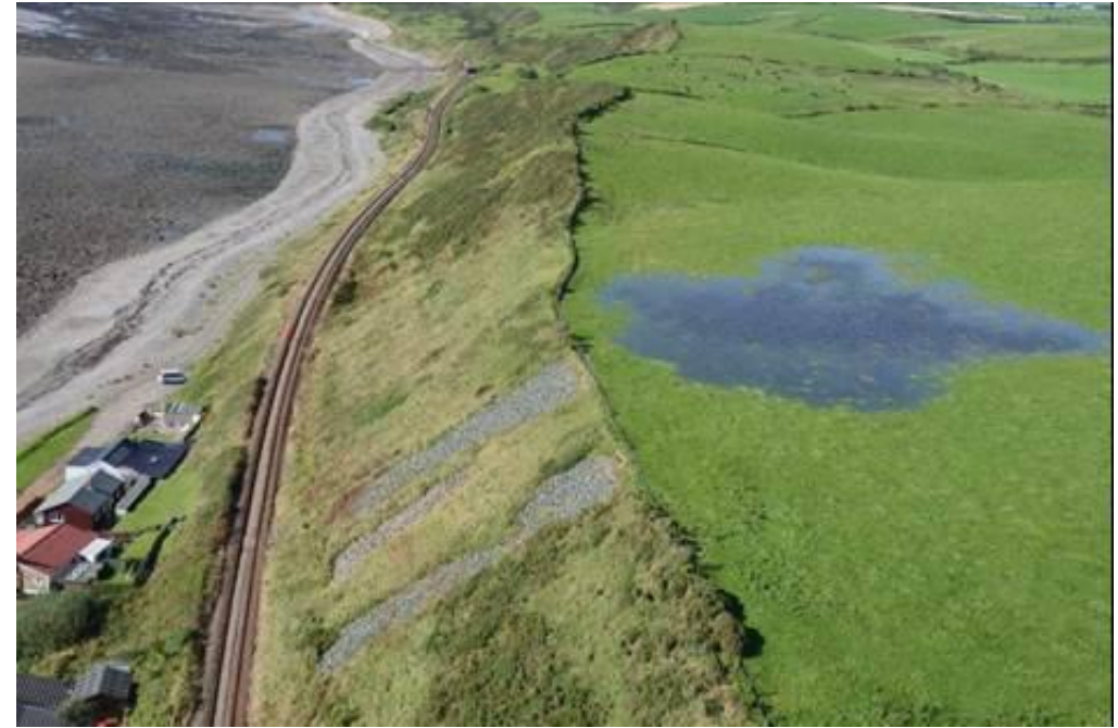
Figure 44 Build up of surface water at the crest of a cutting on the Cumbrian Coast Line in August 2012
