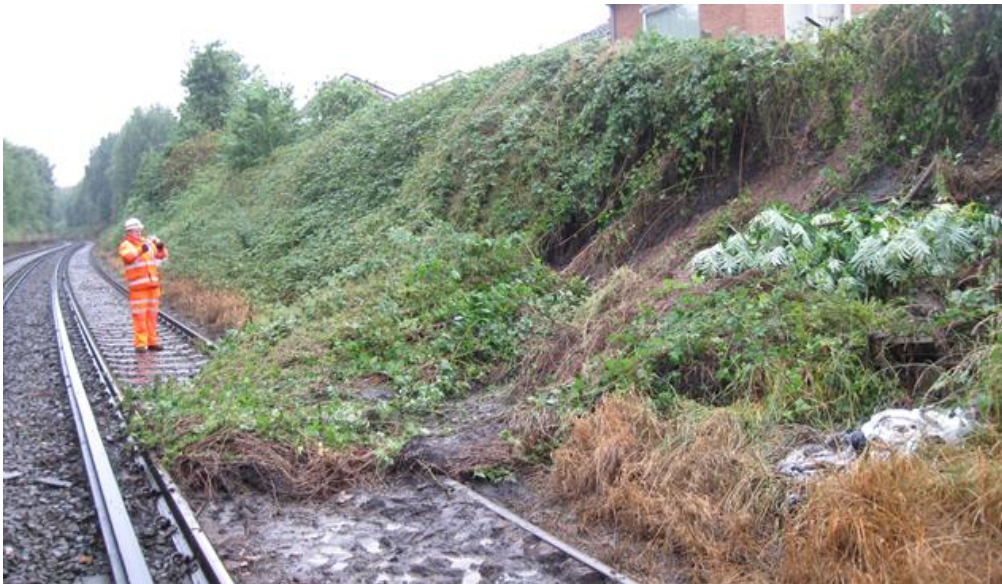
Figure 40 Washout failure at Aigburth in 2010
