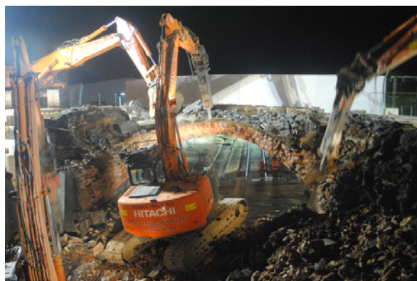
Gauge enhancement works on the Felixstowe to Nuneaton route.
