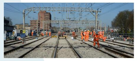
A bridge south of Watford Junction station was demolished and a new one installed enabling line speeds to be increased through the area. As part of a wider £81 million upgrade scheme, old track, signalling and junctions were also replaced.
