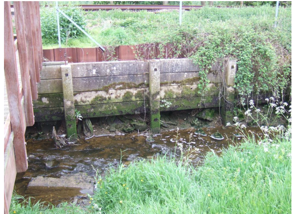
Figure 22 Scour damage at Melton
