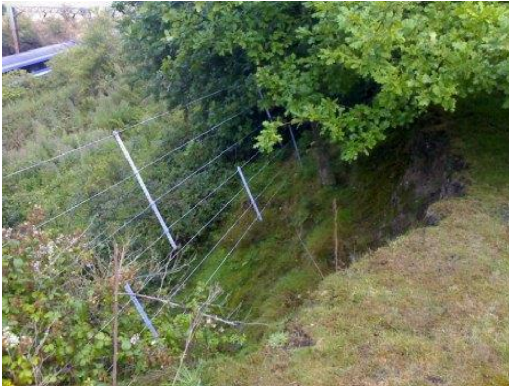
Figure 25 Earthslip at Tumulus cutting
