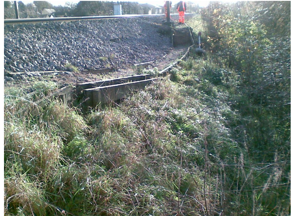
Figure 24 Earthslip at Chelmsford embankment
