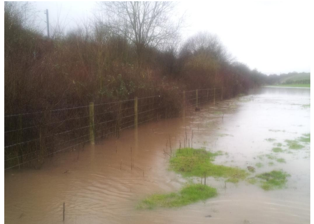
Figure 26 Toe ponding from third-party surface water run-off
