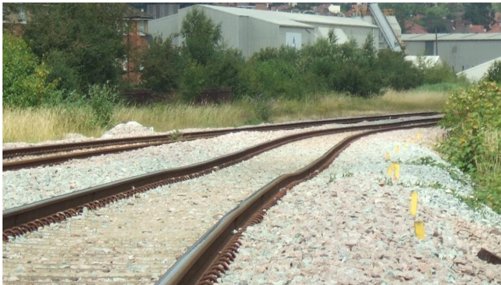
Figure 12 Earthslip at Acton Wells embankment
