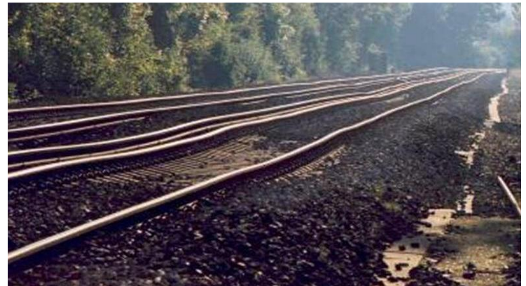
Figure 20 Desiccation/shrinkage risk
