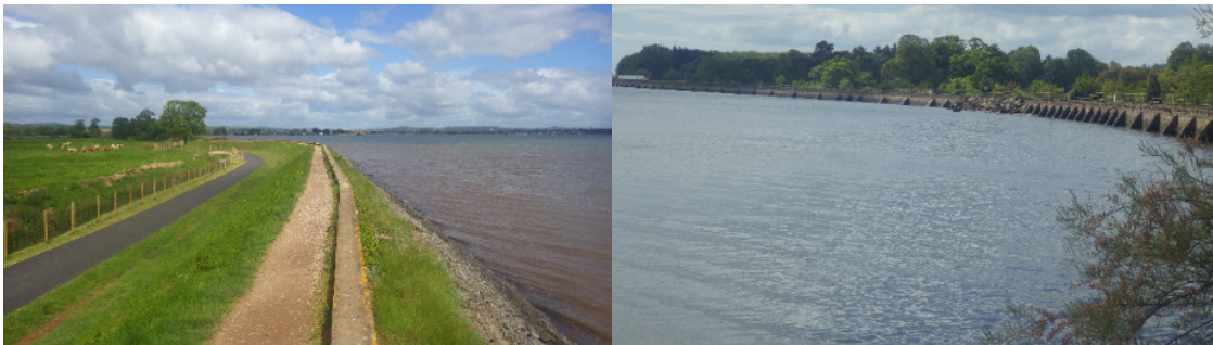
Figure 5-5: Typical defences in Section 1; embankments (northern extent) and buttressed vertical wall (southern extent)
