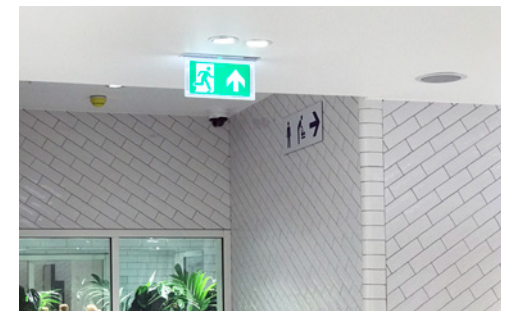
Escape route sign coordinated with light fittings, London Victoria Station. Image: Wendy Hardie
