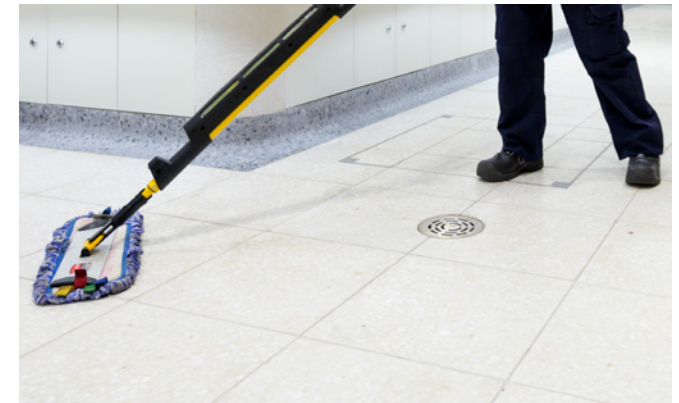
Terrazzo floor tiles (400 mm x 400mm module) with drainage point, access hatches, and contrasting coved skirting. London Victoria WC's. Image: Peter Langdown
