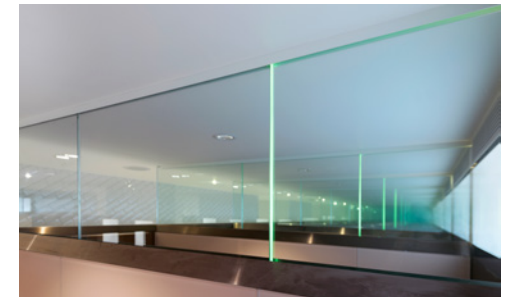
Angled panels atop cubicle walls prevents the concealment of illegal items, London Victoria WC's. Image: Peter Langdown
