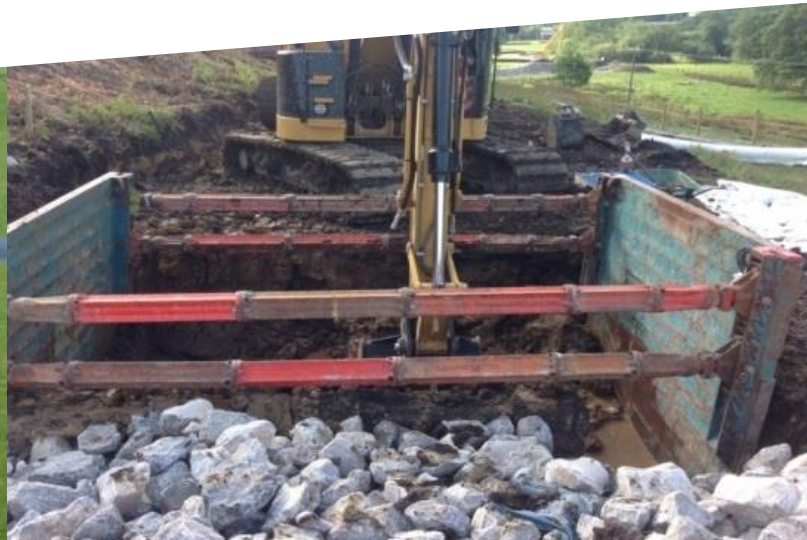
Below: Slope repairs on a cutting beneath a natural depression where water accumulates (left) and construction works taking place with temporary support to excavation (right)
