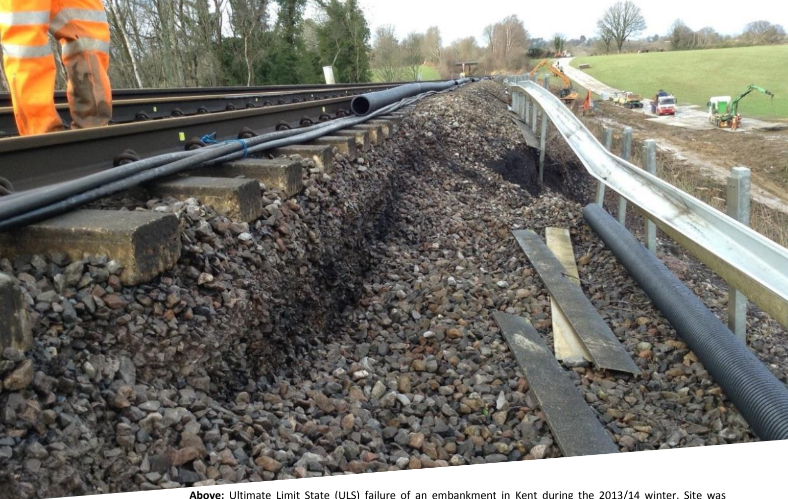
Above: Ultimate Limit State (ULS) failure of an embankment in Kent during the 2013/14 winter. Site was exposed to high maintenance frequency as a result of Serviceability Limit State (SLS) failures over several years.
