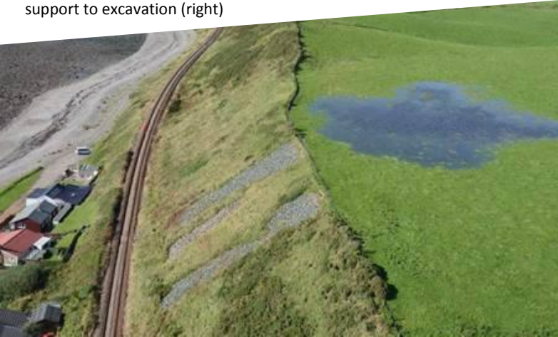
Below: Slope repairs on a cutting beneath a natural depression where water accumulates (left) and construction works taking place with temporary support to excavation (right)
