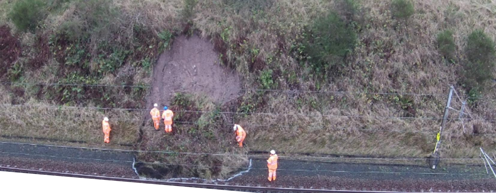
Above: Rapid failure of a soil cutting at Murthat in Scotland on the West Coast Main Line (Nov 2015). Asset showed no evidence of failure prior to slumping towards the track after a period of relatively normal rainfall. Failure identified by the driver of a passenger train travelling at 125mph.
