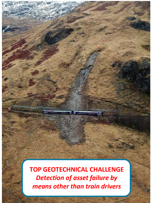
Above: Passenger train derailment on the Fort William to Mallaig line (January 2018) following the collision with material from a debris flow. Originating from the adjacent mountainside the debris flow mobilised rapidly and was encountered by a passenger train with the driver unable to stop in advance of the failed material.
