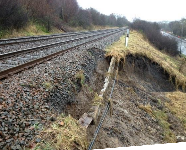
Above: Typical earthwork failures within the NR database that was used to undertake a correlation with weather data.
