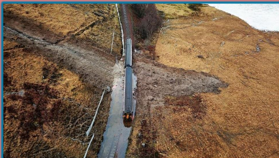
Below: A rapid debris flow failure from an adjacent hillside which caused a passenger train to derail. The detection of such rapid failures is our top geotechnical challenge, recognising we cannot instrument all hazardous or all high consequence locations (i.e. deployment of technology has to be risk based).
