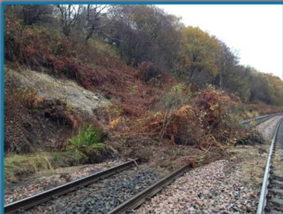
Above: Example of a rapid failure within a soil cutting in response to short duration high intensity rainfall event and sign advising lineside operatives that a cutting slope contains a live monitoring system.
