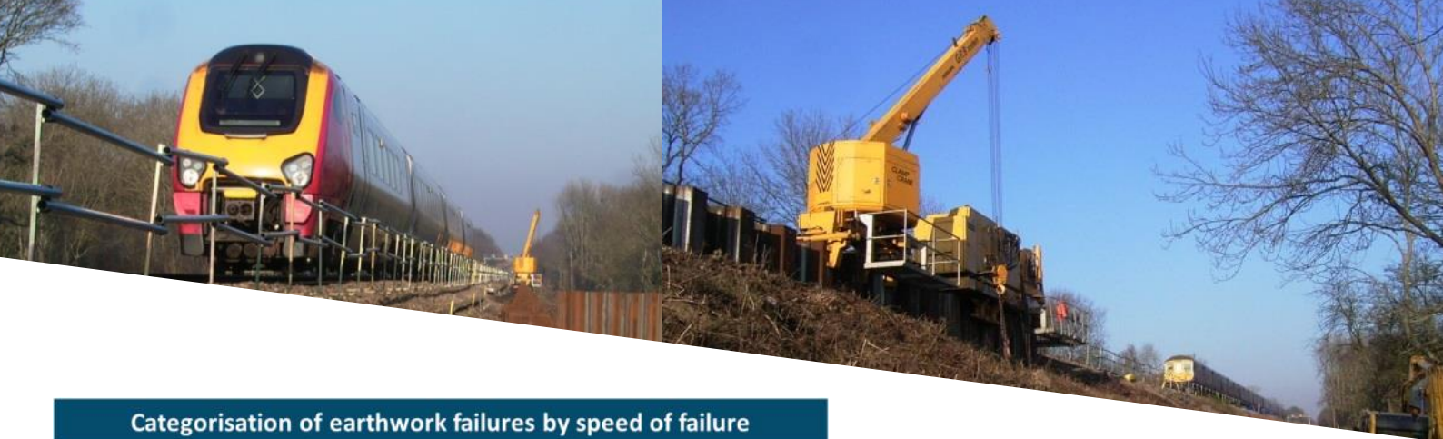
Above: Construction of a sheet pile wall at the crest of an embankment on the Brighton mainline in CP4 using the silent and vibration-less GIKEN technique.
