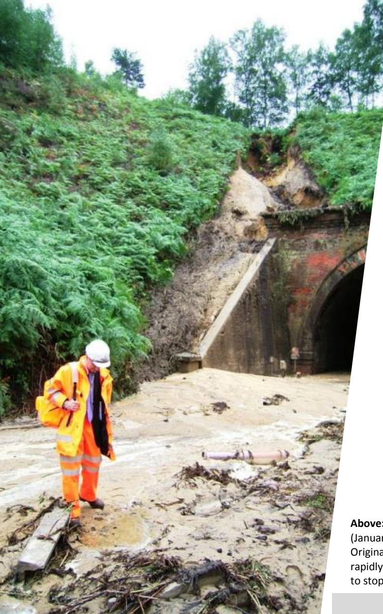
Left: Washout at Foxhills Tunnel following a deluge of 90mm of rainfall within an 8 hour period (August 2006).
