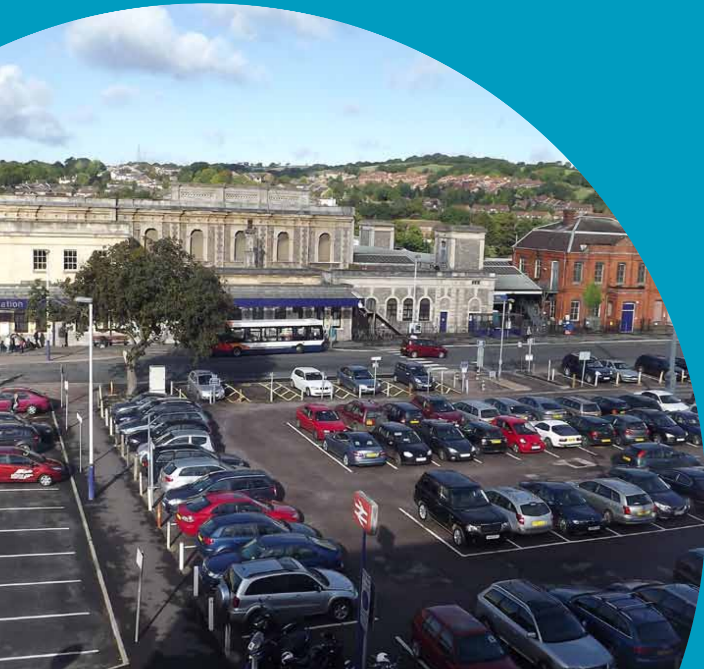
Photograph of existing site and station
