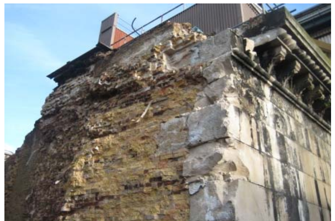
Some of the bridge stonework will be retained on site for reuse in the new station.
