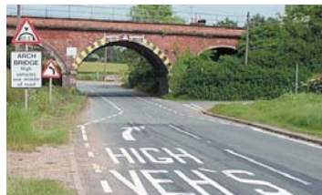
White lines on the road indicating the extent of the signed vehicle height limit
