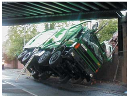
A waste lorry on its side following a bridge strike
